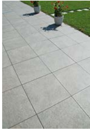
Pose joint croisé
